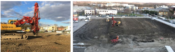
Figure 4. Rapid impact compaction (R.I.C.) for brownfields.
