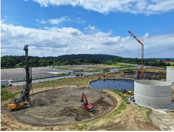
Figure 5. CMC execution for the tank foundation.
