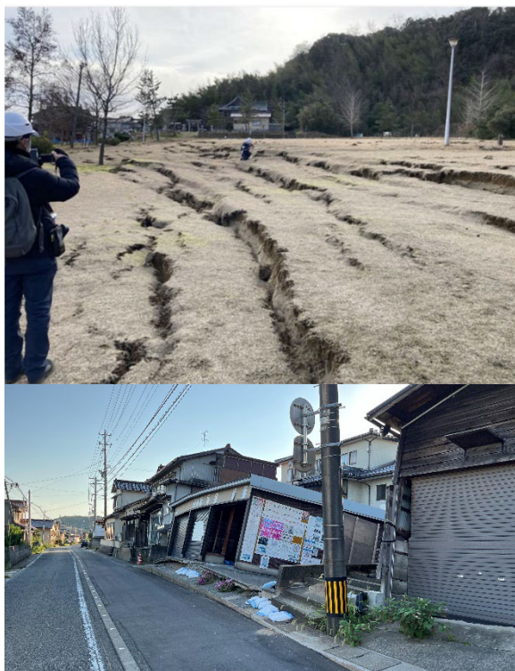
Figure 2. Damages from liquefaction in Uchinada Town
